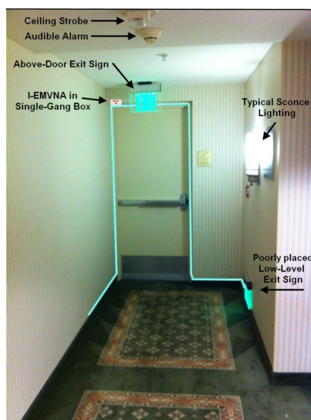
Typical End-of-Corridor Hotel Exit (normal operating conditions no fire/smoke)
